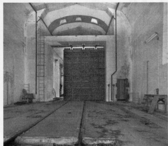
The shock-absorbing sliding doors at the Söderhamn converter station in 2006. Photo by Nick Catford
